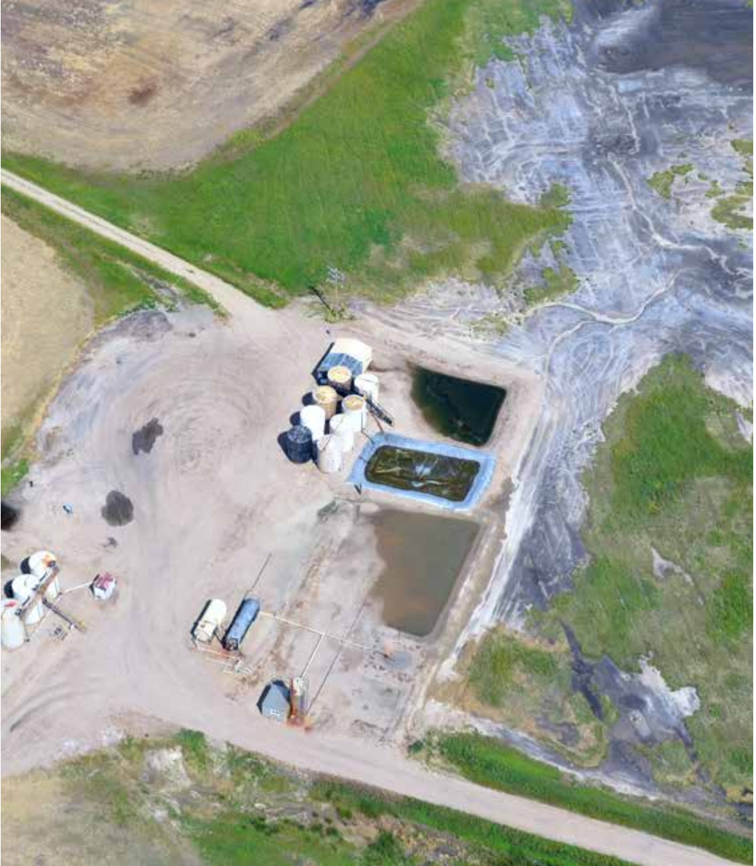
Leaching salt damages farmland up to 500 feet from oil facilities as seen in this site in Bottineau County in north-central North Dakota. Photo courtesy of Northwest Landowners Association.
