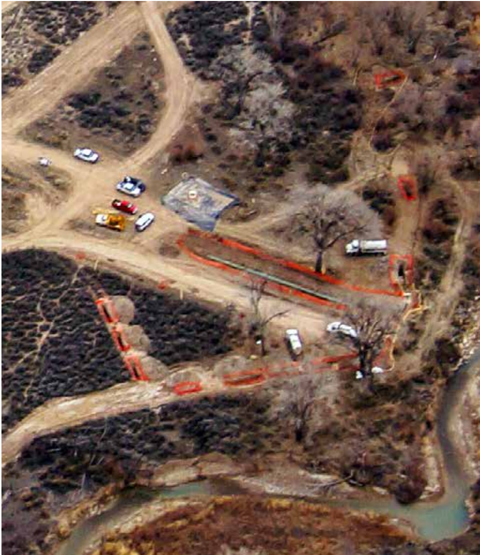
Vacuum trucks collected over 60,000 gallons of hydrocarbon material and 5,400 gallons of oil from the Parachute Creek gas plant leak in Garfield County, Colorado. Cancer-causing benzene was detected in the groundwater and in the creek. Photo courtesy: Ecoflight, ecoflight.org.
