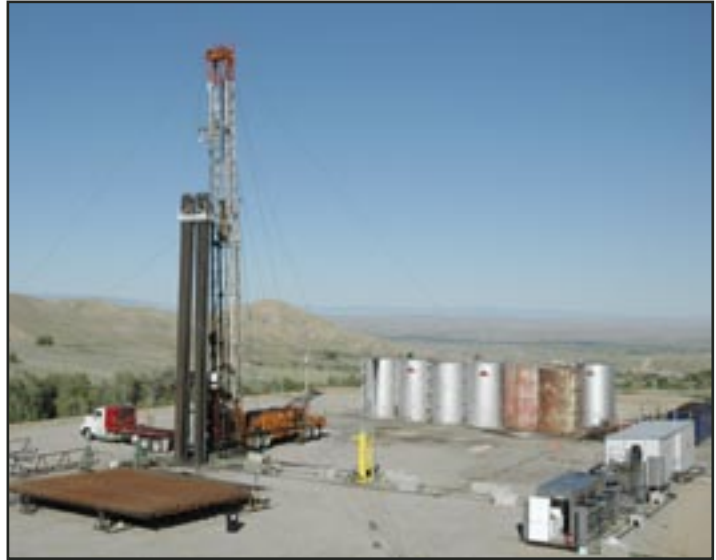
Tight sands drilling operation near Clark, Wyoming.
