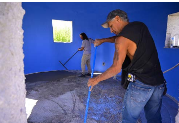
Jason Mackie and Leo Bear apply a self leveling flooring in a model home.
