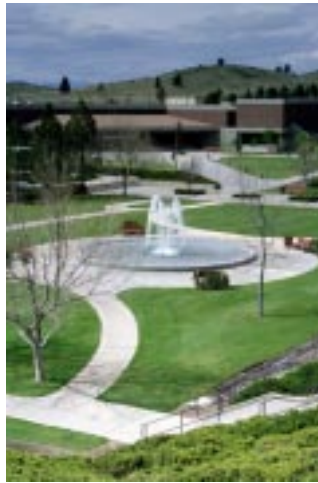
The Oregon Institute of Technology has been using a geothermal district heating system since 1964. Today, the system heats 11 buildings.
